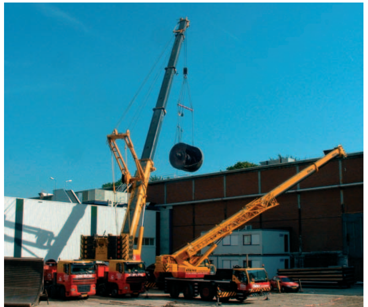
Removal through the production hall's roof.
