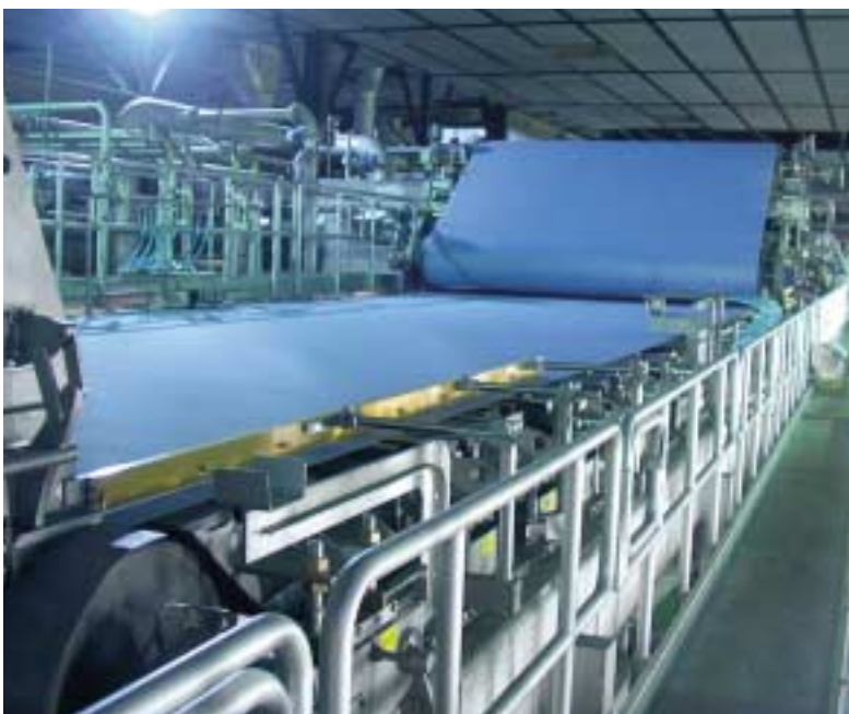
The refurbished KM3
