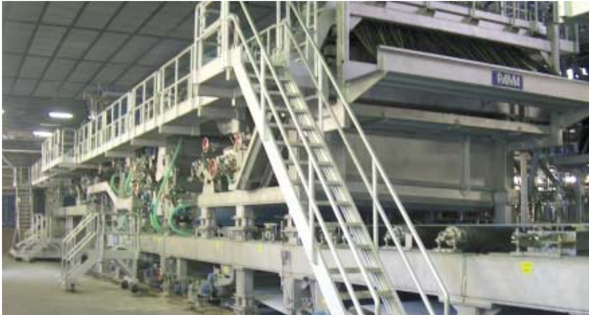
The refurbished KM3
